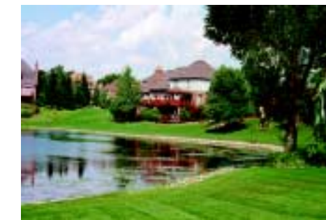
Wet Detention Basin
