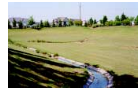
Dry Detention Basin
