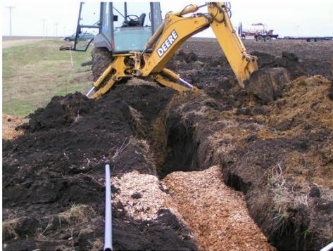
A woodchip bioreactor being installed in Minnesota.
