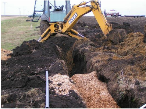
A woodchip bioreactor being installed in Minnesota. (Minnesota Dept. of Agriculture, University of Minnesota Extension)
